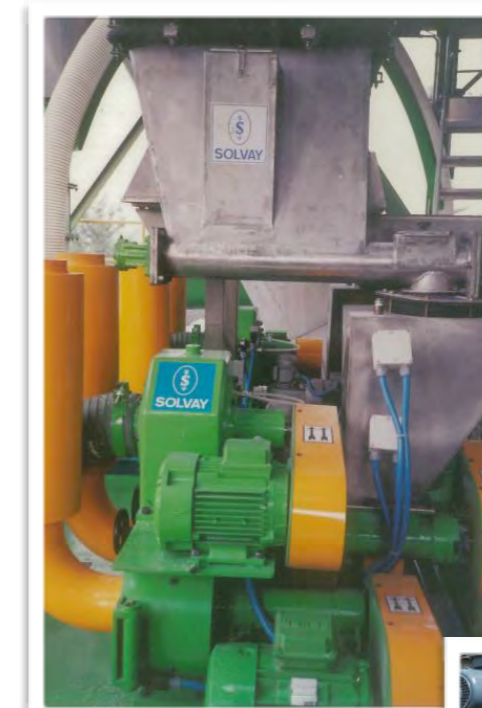
STM Serial No. 1. Reggio Emilia Incinerator, Italy
